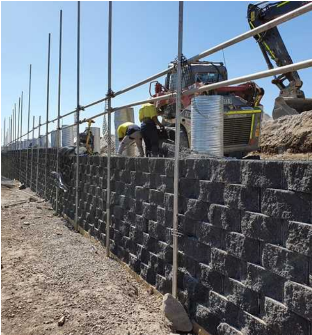
Plate 4. Installation of the Keystone TW3 wall with corrugated pipes for noise barrier foundation
