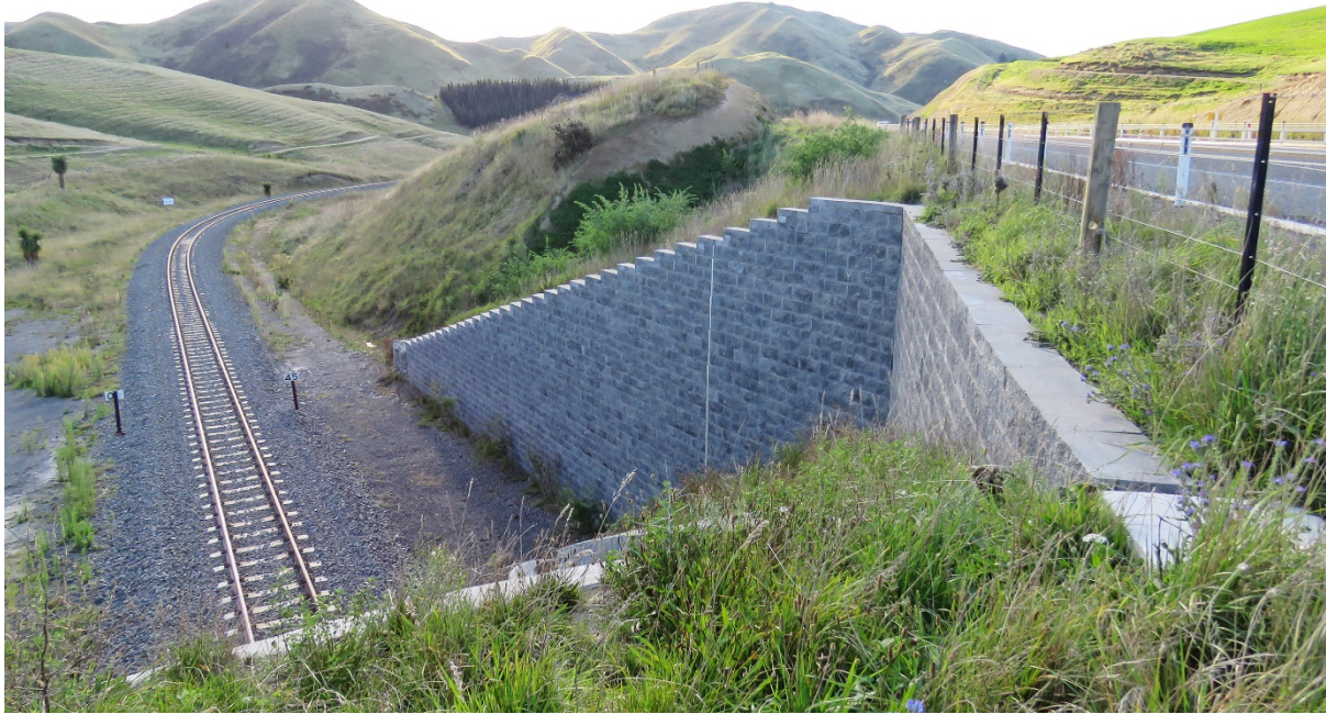
Plate 2. View of the Keystone TW3 wall at Dashwood with the slip joint visible
