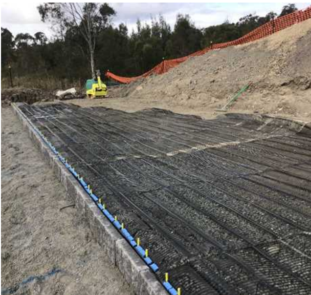
Plate 3. Construction of Keystone TW3 wall for Maitland Hospital
