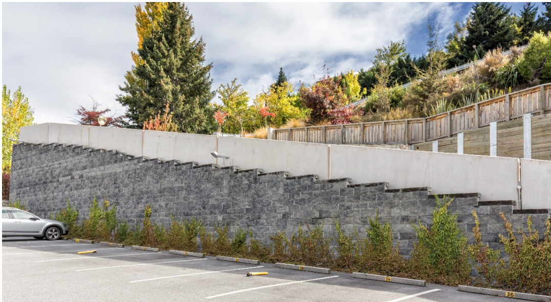
Plate 1. View of the Keystone TW3 wall at La Residence Du Lac
