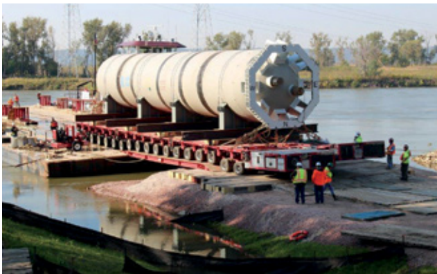
Pressure vessels and other plant components were transported from river barges to the heavy laydown area along a heavy haul road stabilized with Tensar TriAx TX160 Geogrid.
